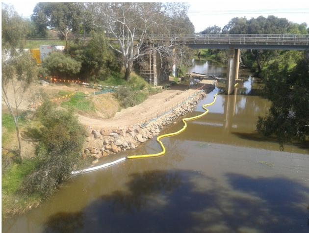
The new bridge will be at the ten year flood level or about three metres above water on normal flows in that area. It will be a timber deck bridge supported by steel framework and piles. Once construction has finished the cofferdam will be removed.
