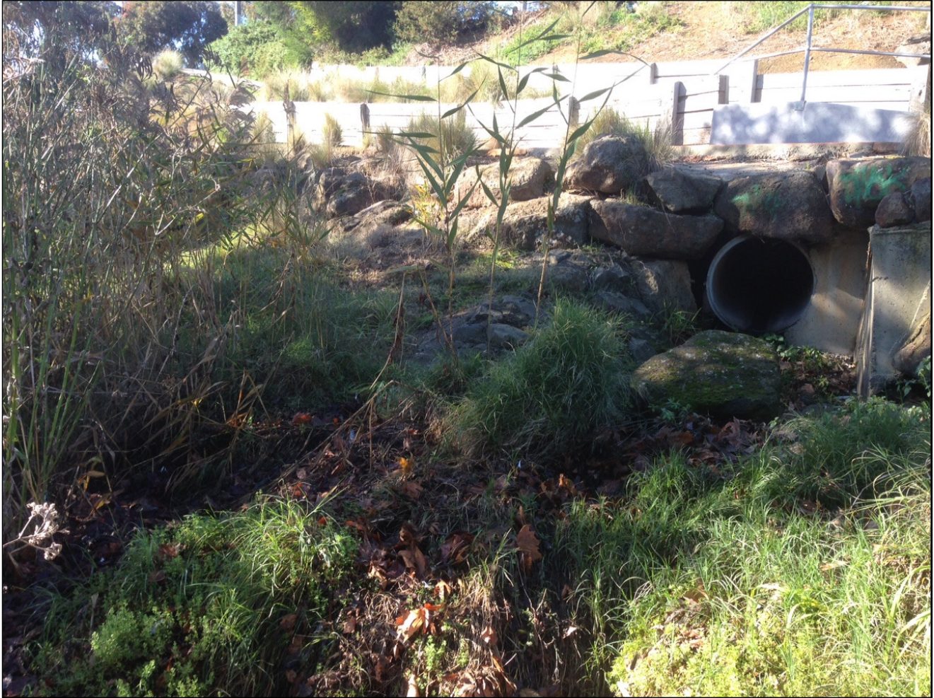
Bridge St Drain
