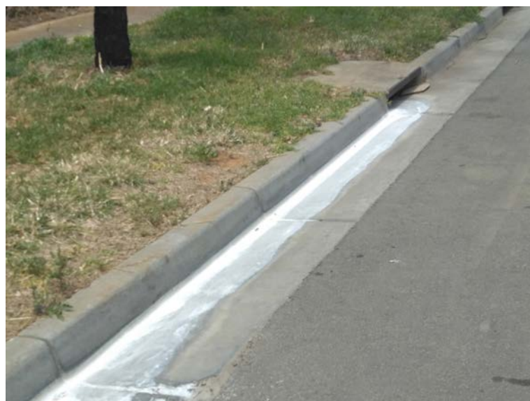
Figure 29 Pollution discharging from a local business in the Maltby industrial area. The pollution event was reported to EPA which resulted in action being taken to mitigate the impacts downstream.
