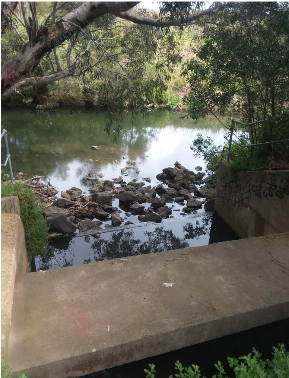
Figure 5 Maltby bypass stormwater outlet
